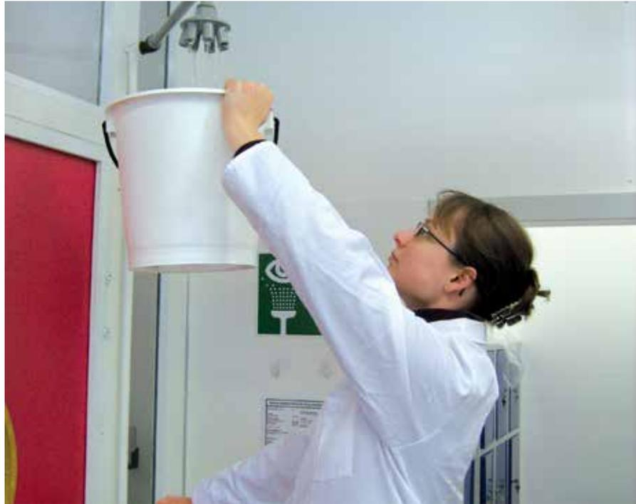
Labour-intensive water exchange at every terminal tapping point. A common, but ineffective and expensive solution to ensure proper operation in a building.
