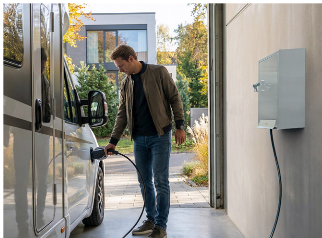
Power supply for private use – securely protected against access by unauthorised third parties.
